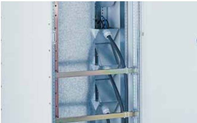
Cable connection compartment at the rear with one cable gland box per functional unit, internal separation Form 4 Type 7 acc. to BS EN 60439
