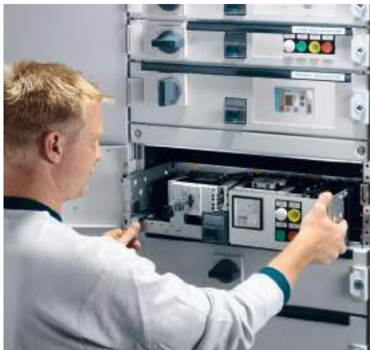
The mechanical coding of the withdrawable unit prevents any confusion of withdrawable units of the same size.
