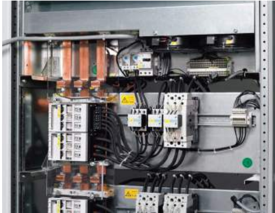
The capacitor assemblies can be used in choked or unchoked condition.
