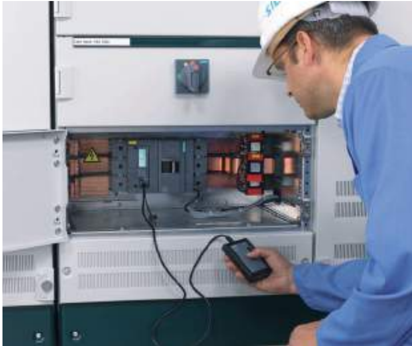
Fixed-mounted design with 3VA circuit breaker
