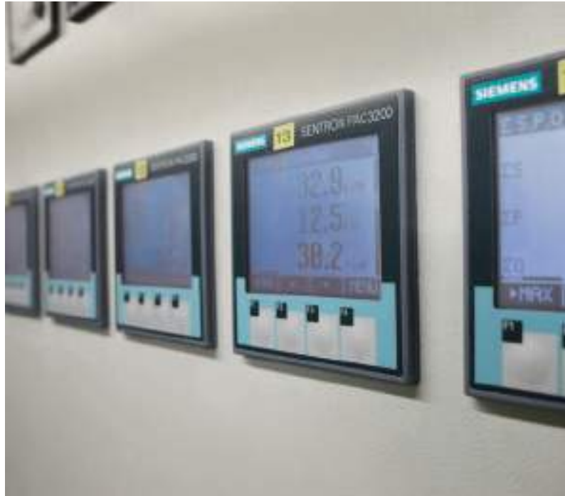
Communication-capable measuring devices 7KT PAC
