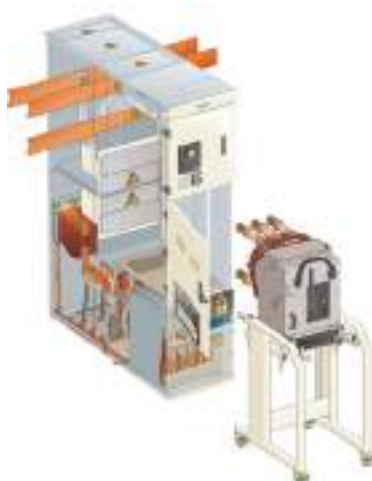
Fig. B28 Example of functional unit architecture with compartments, favoring service continuity
