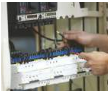
Fig. E30 Assembly of a final distribution switchboard with fixed functional units (Prisma G)
