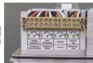
(b) Contacts of the DGPT (cover removed)
