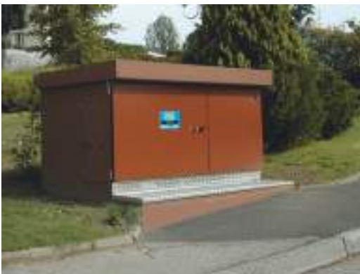
(b) Half buried non walk in type substation
