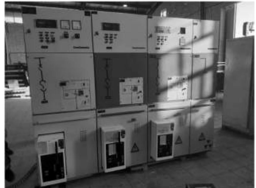
MV/ Compact type 24 kv
